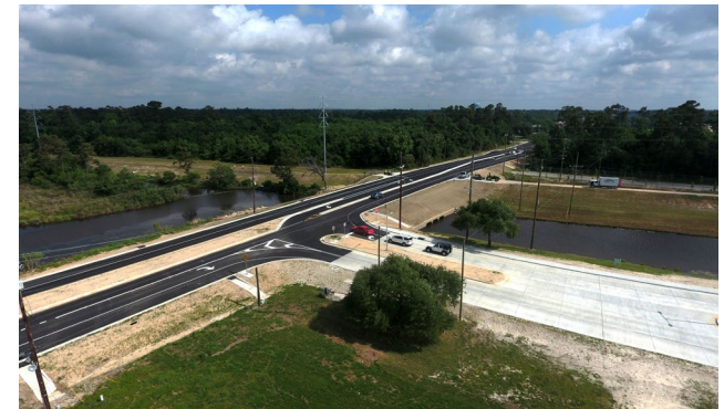
The addition of a bike path provides accessibility and safety for pedestrians while the drainage improvements reduce the risk of road flooding and water hazards for motorists.
